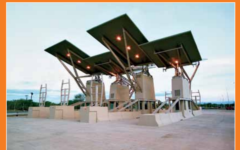
ABOVE: Baobab Toll Plaza, on the N1 Highway between Musina and Makhado, Limpopo, was designed by Mathews & Associates Architects. The architects derived conceptual inspiration from the baobab tree, which is indigenous to much of Africa, and endemic to Limpopo. It is the emblem of the province.
